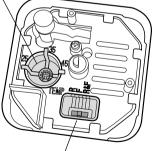
The regulating function is adjusted here. **F** - Floor thermostat **R** - Room thermostat **R&F** - Room and floor thermostat
