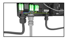
**Note:** If not routing the heat trace directly, use the cold leads connected to the heat trace from the junction box for the heater wiring to the unit.
