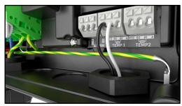
f. Tighten the cable gland cap by rotating clockwise applying the recommended torque.
